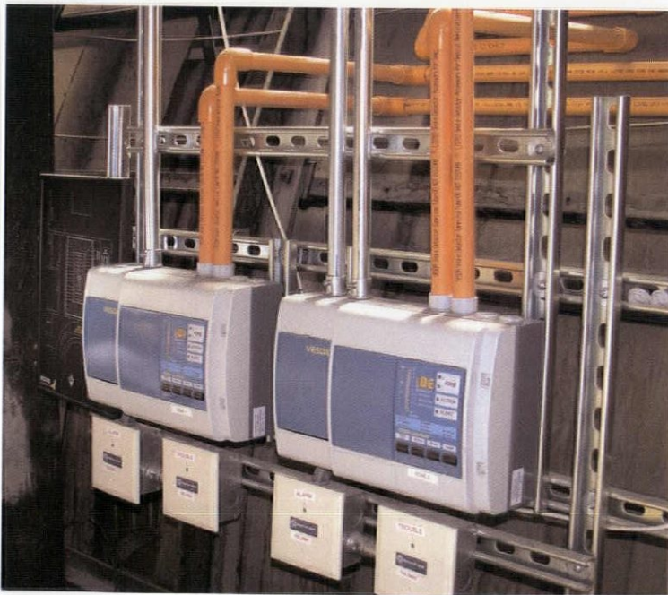
PREVIOUS The Colorado State Capitol Building is recognized as both an historic building and an important symbolic icon of state government. LEFT The Vesda air sampling system OPPOSITE The glass doors were fabricated with a water jet cutter to follow the profile of the historic marble wainscot rather than attaching them to the walls.
