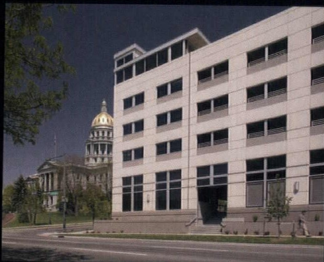
James Merrick State Parking Facility, Denver, CO Architect: Carl Walker Inc./Shears Adkins
