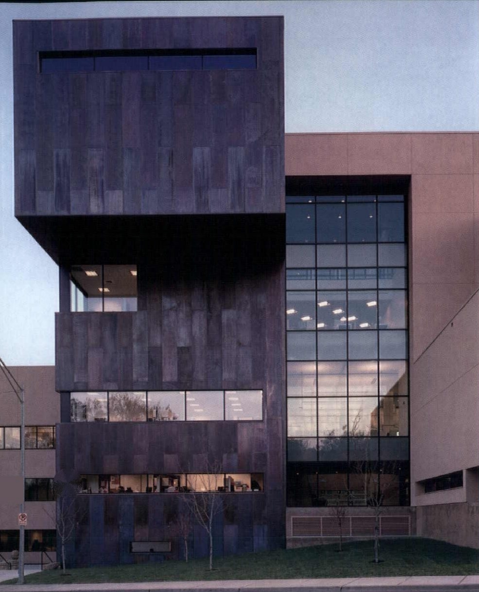
Antoine Predock's Robert Hoag Rawlings Public Library in Pueblo was designed in collaboration with Denver's Anderson Mason Dale Architects.
