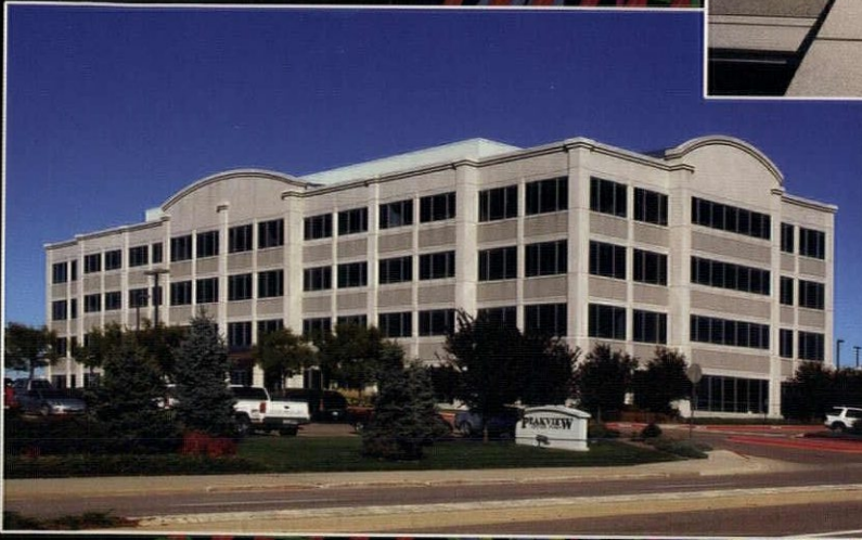
Peak View Office Building
