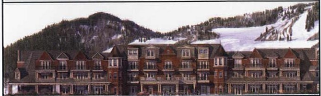
Grand Aspen Lodge — In Progress O'Bryan Partnership
