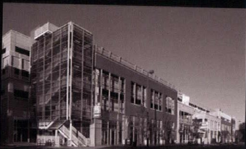
Clayton Lane Parking Facility Cherry Creek North District, Denver, CO
