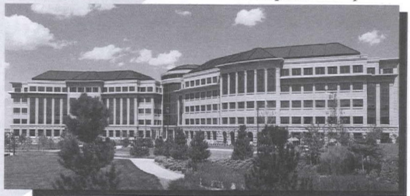
Owner: Starz Encore General Contractor: The Wertz Company Architect: Barber Architecture Engineer: S.A. Miro
