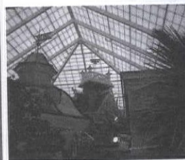
CRÉME DE LA CRÉME CHILDCARE LONE TREE, COLORADO Kabwall - 70 ft. x 40 ft. hipped self-supporting translucent skylight
