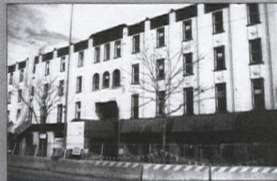
Northern Hotel - Fort Collins
