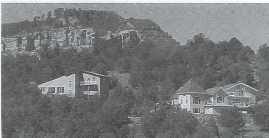
Designing on the West Slope requires sensitivity to hillside environment
