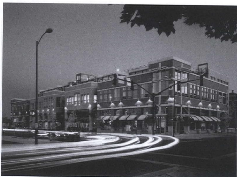
Honor Award for Architectural Excellence: 15th & Pearl Parking Structure. Boulder, CO. Architect: RNL Design and Shears & Leese
