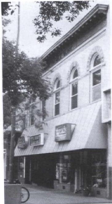
Trimble building before renovation
