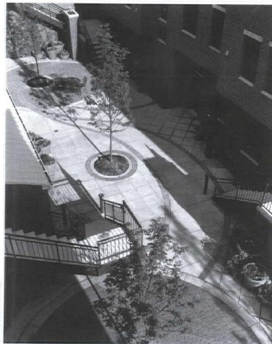
Partial exterior view of Mawson Block. Architect: RB+B Architects, Inc.
