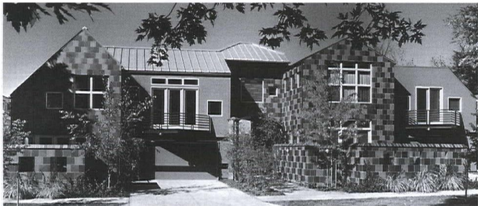
421, 423, 425, 427 Detroit Street A mural of Egrets flying overhead is painted on the underside of the archway leading to the entry courtyard.
