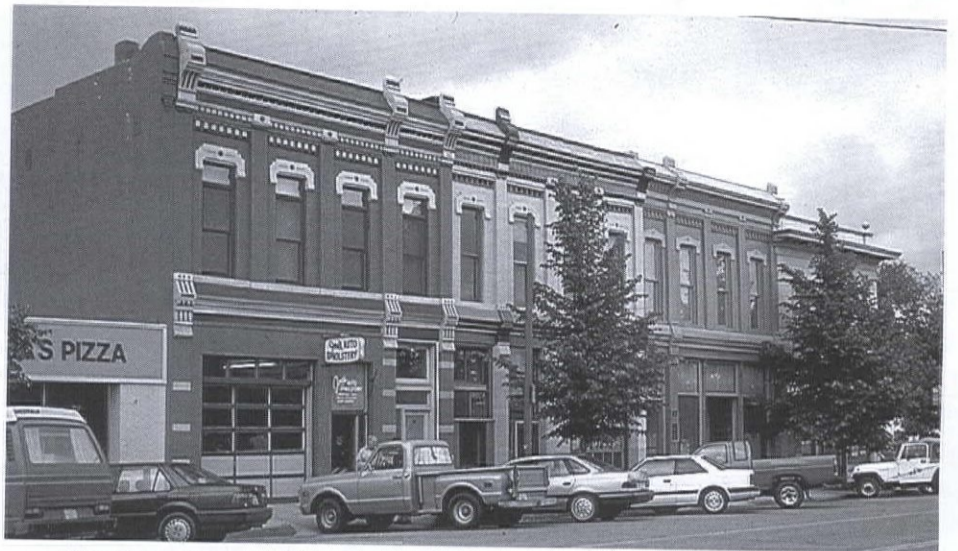
After: Restoration work followed the Old Town Design Guidelines. In some cases, missing storefronts were reconstructed. In others, later uses were retained and designs were developed to enhance the historic character while retaining future restoration options.
