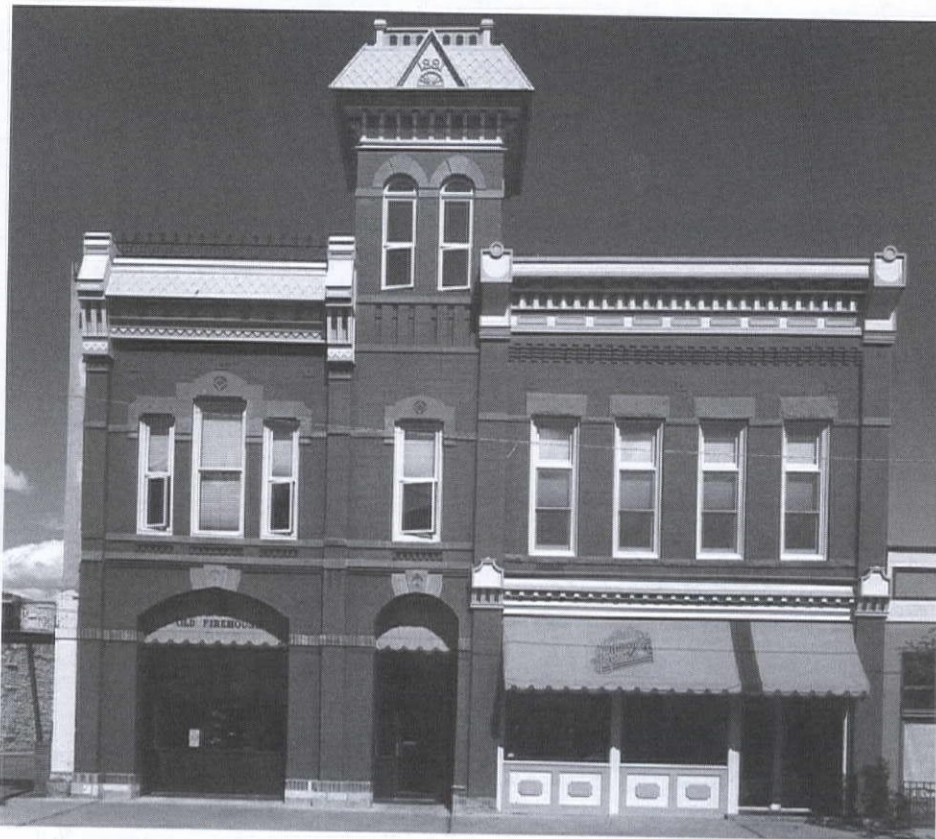
A preservation approach was developed that not only restored the structures to their previous glory, but also helped secure federal tax credits for the owner.
