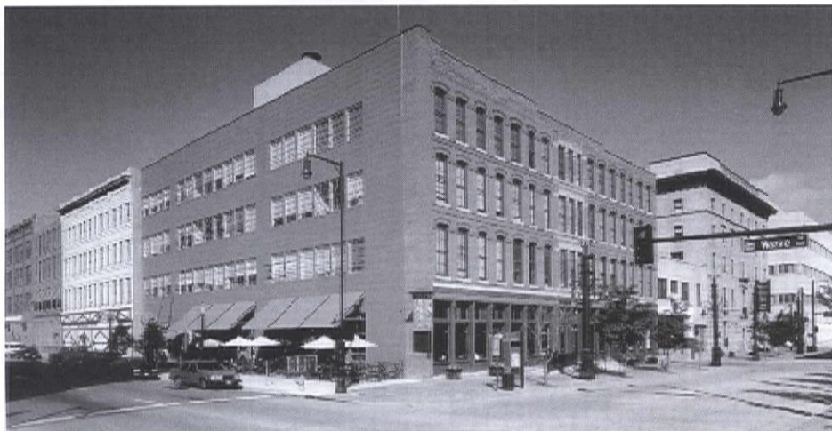
Mercantile Square/Tattered Cover Bookstore/Wines Off Wynkoop, Denver. Architect: David Owen Tryba Architects, Design Honor Award winner.
