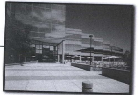
Lucent Technologies Associate Service Court Addition
