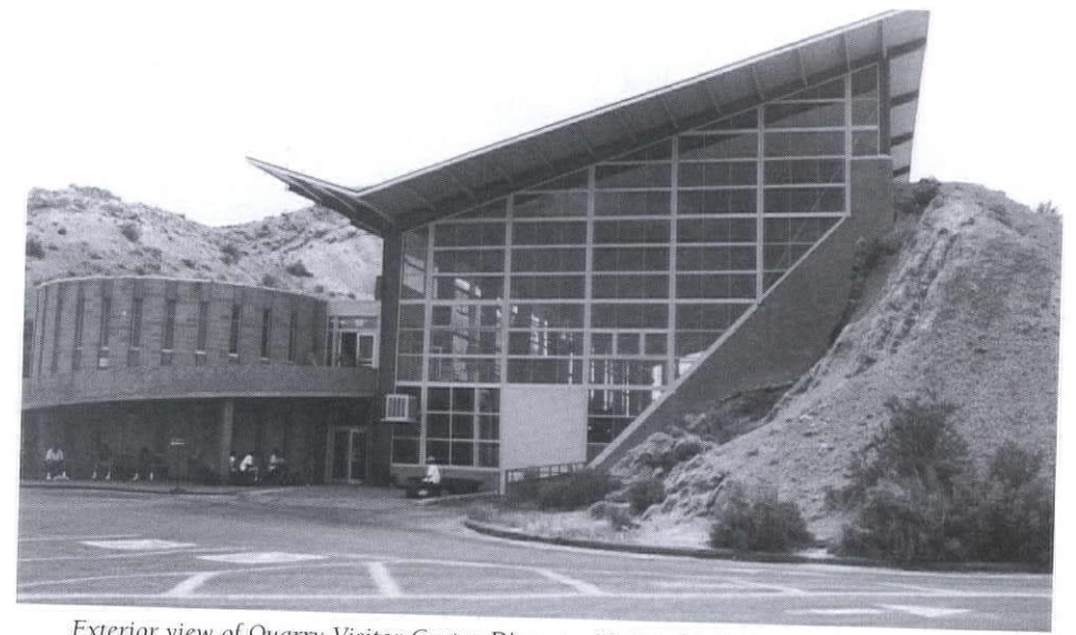
Exterior view of Quarry Visitor Center, Dinosaur National Monument.
