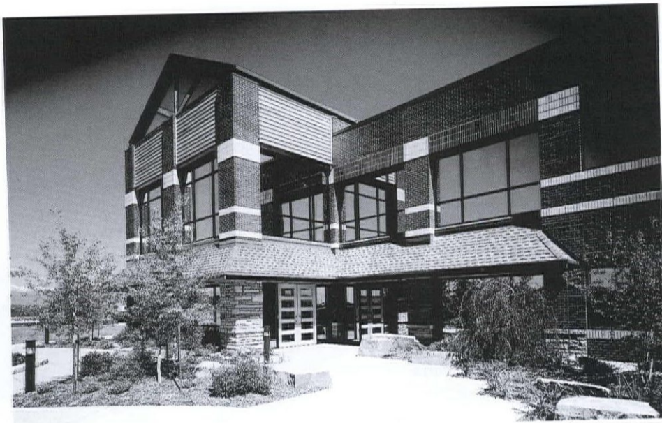
FDC Office, Phase I. Loveland, Colorado. Architect: The Neenan Company.
