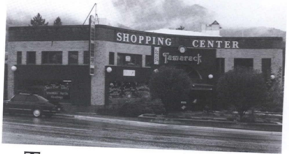
Tamarack Building before remodeling project.
