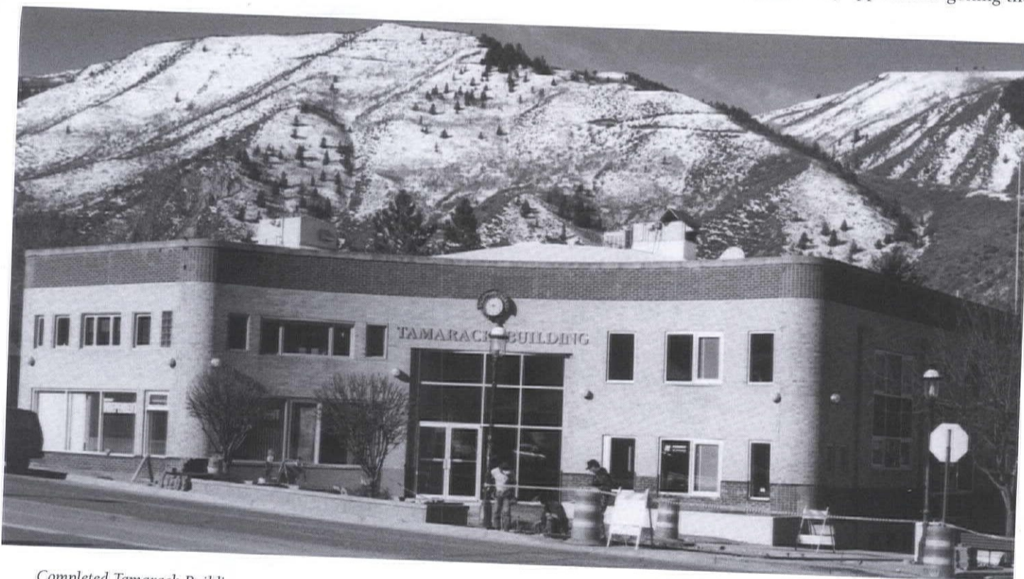
Completed Tamarack Building remodel project.
