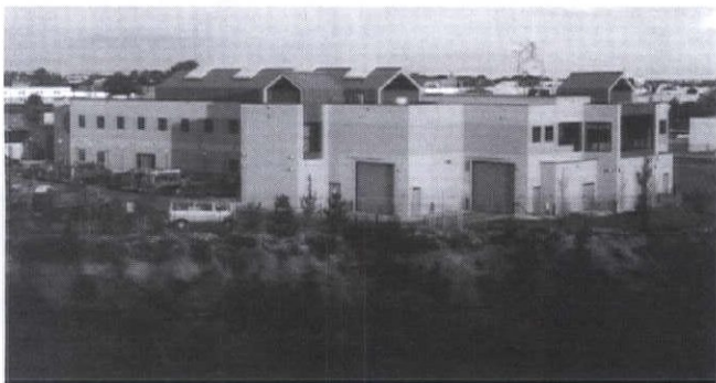
Colorado Springs Utilities Gas Department - Operations Bldg. Addition & Remodel. 1995 Merit Award - AIA Colorado South Chapter
