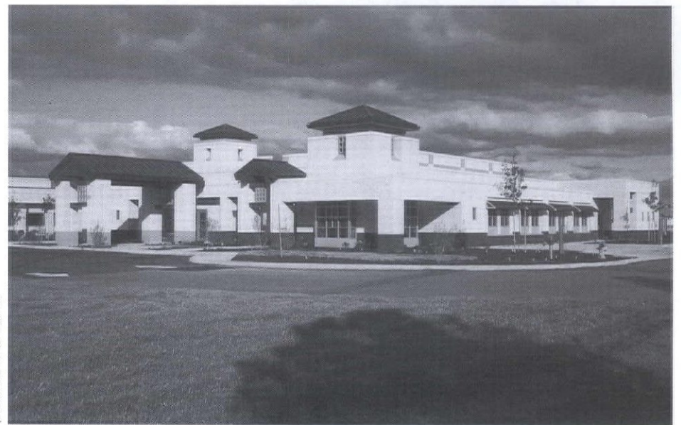
Cypress Surgery Center, Visalia, California. Architect: Boulder Associates.
