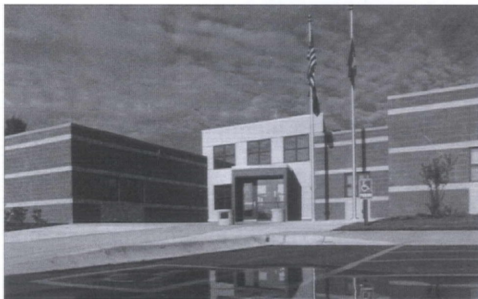
The Nebraska Correctional Youth Facility is laid out in a modified campus plan. Classrooms face into the secure courtyard, and the buildings themselves from most of the security perimeter.
