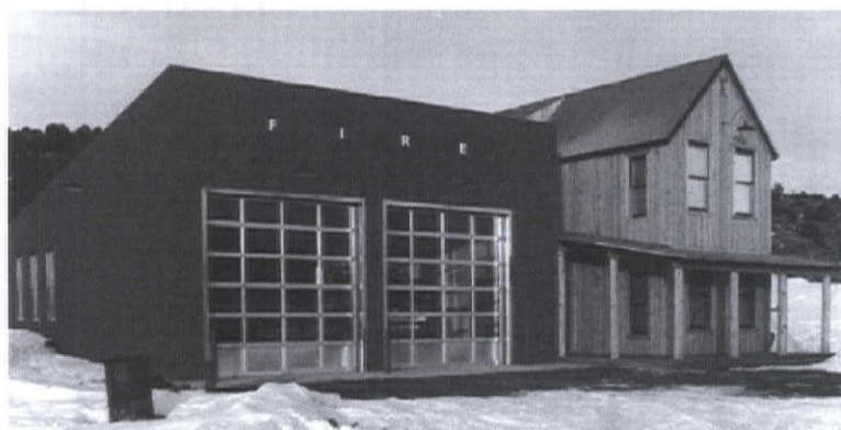
Carbondale Rural Fire Station - Honor Award 1995
