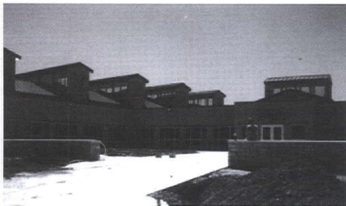
The Fine Arts Building by Anderson Mason Dale of Denver with R. M. Bell & Associates, Durango.
