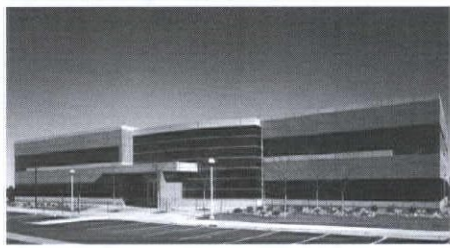
Calcon prides itself on its ability to build unique structures.
