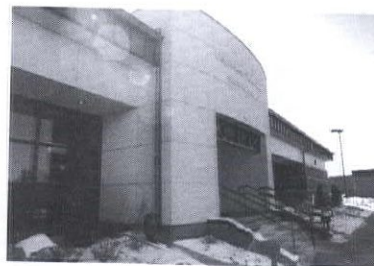
Ent Federal Credit Union Galley Branch
