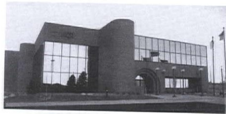
Association of Christian Schools International Headquarters Building
