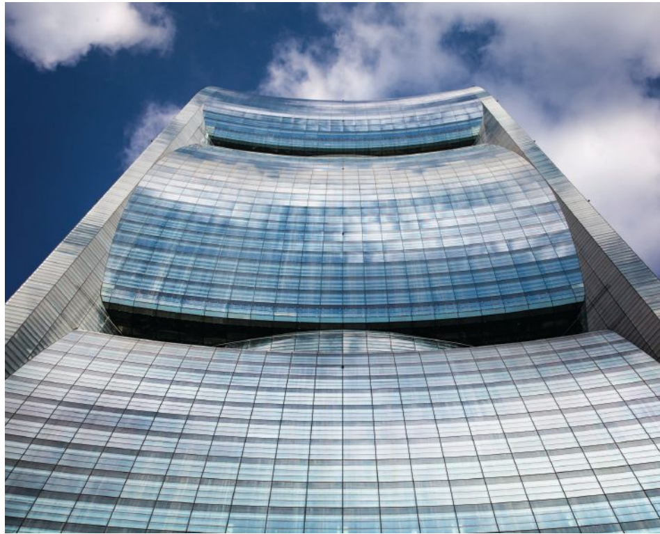
Completed with SOM in 2013, Pearl River Tower in Guangzhou, China, incorporates wind turbines for on-site electricity generation that shape its distinctive cinched profile. TIM GRIFFITH
