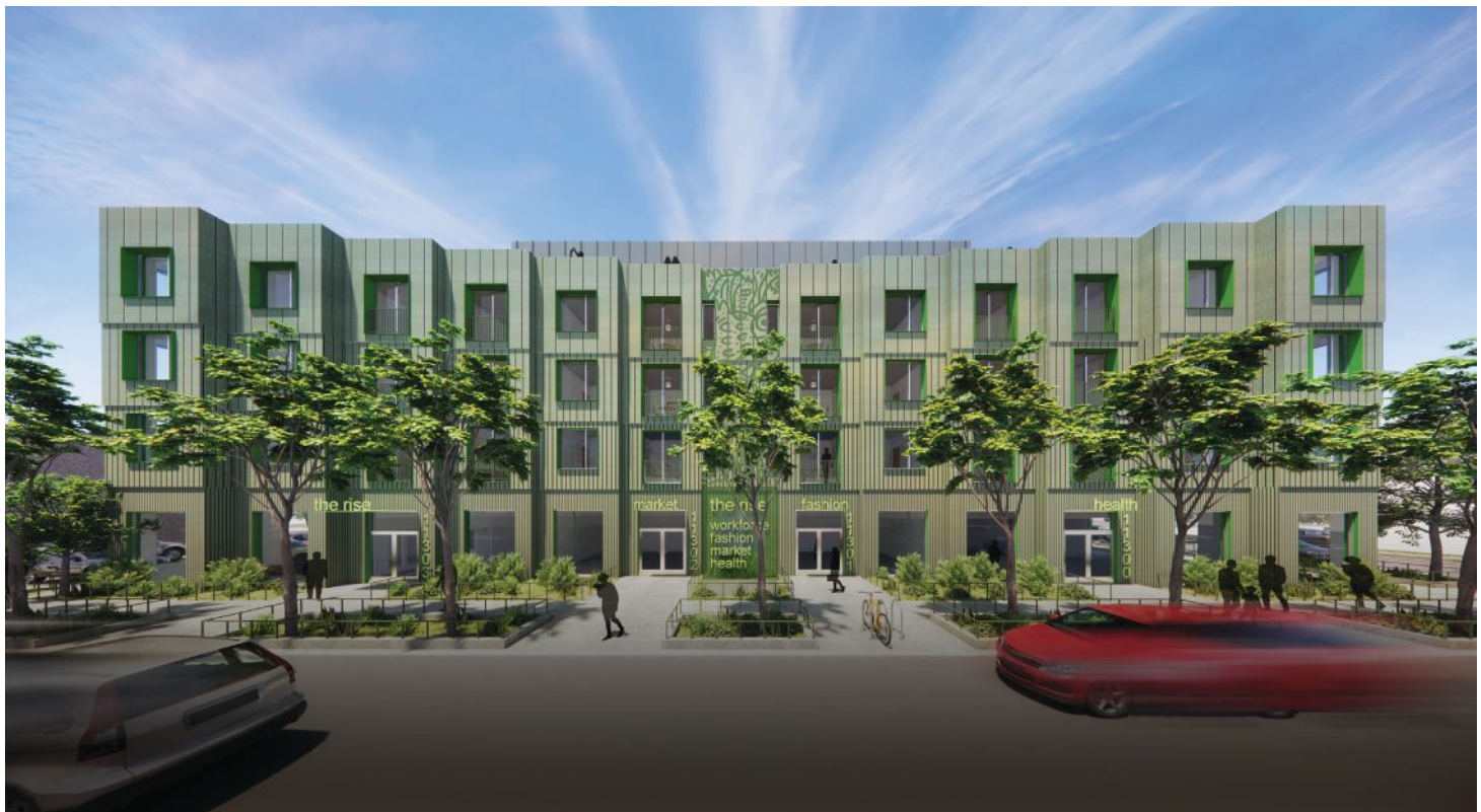
At top: Morgan Park Commons, a mixed-use development on Chicago's Far South Side, is transforming a lot that has sat vacant for more than a decade. RENDERING BY LAMAR JOHNSON COLLABORATIVE At bottom: Located in Morgan Park, The Rise is a five-story market rate and Department of Housing project with retail functions at the ground floor. LATENT
