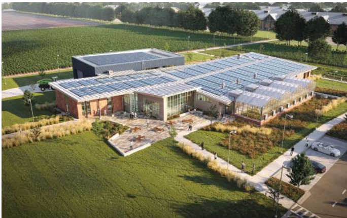
Legat Architects recently completed Heartland Community College's Agriculture Complex, a 29,500-square-foot building that is on track to become Illinois' first native net-zero community college building. The term "native" means that the building was designed to produce at net-zero energy levels immediately upon completion or within the initial 18-month reporting period mandated by the Illinois Clean Energy Community Foundation.
