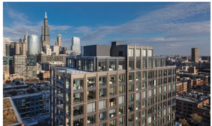
The Chicago office of Lamar Johnson Collaborative (LJC) , in collaboration with interior design firm KARA MANN Design (KMD) , has announced the completion of Embry, a 58-unit, 16-story luxury condominium building at 21 North May Street in Chicago's West Loop.
