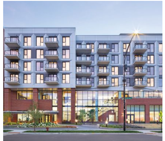
The North Sheffield Development & Edith Spurlock Sampson Center, designed by the team at RATIO Design , pays homage to the first African American U.S. delegate appointed to the United Nations. The new, mixed-income residential building in Lincoln Park for the Chicago Housing Authority and PIRHL transforms a '60s-era senior development into a revitalized community with vibrant amenities.
