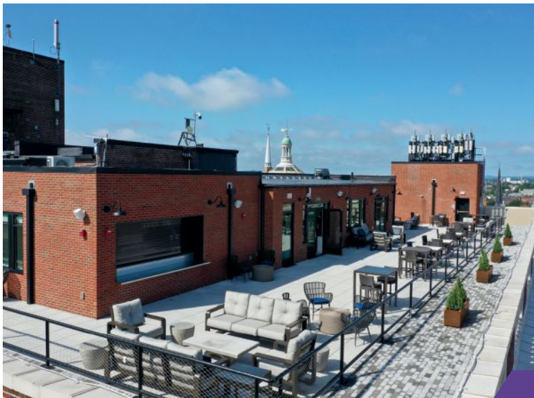
Credit: WINNER/Renovation / Larson Lightning Protection/ BBEC
