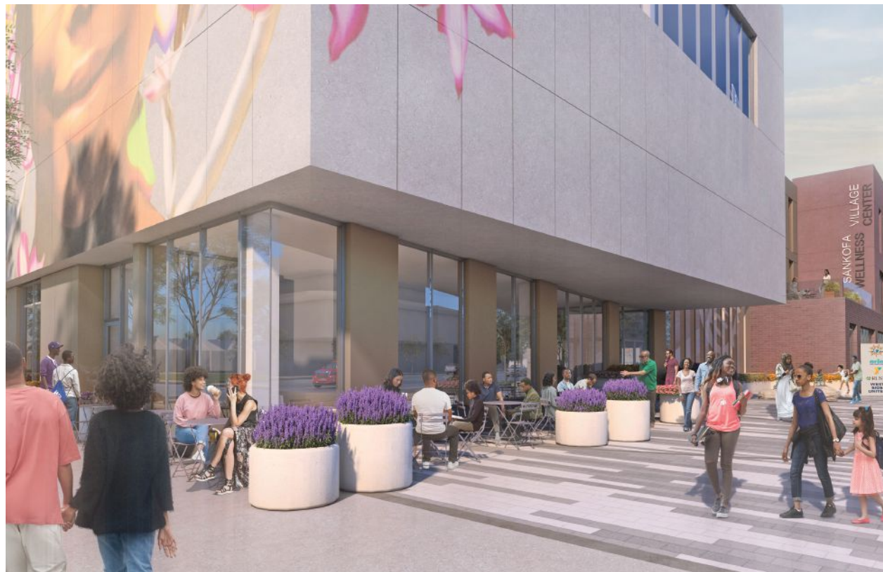
IMAGES BY MOODY NOLAN, ARCHITECT OF RECORD, AND THIRD ENTITY, ASSOCIATE ARCHITECT
