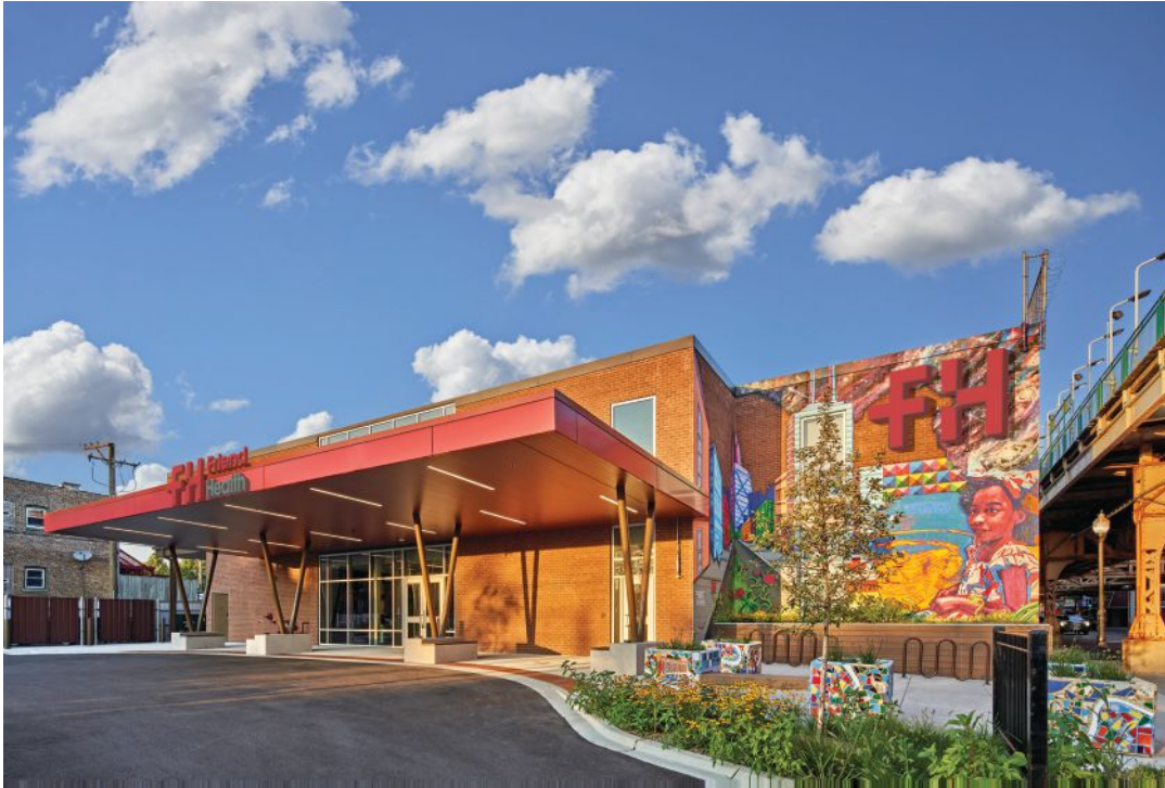
Moody Nolan announced the completion of the Friend Family Health Center, a multi-use medical facility spanning three blocks in Woodlawn on Chicago’s South Side. Moody Nolan renovated the space that was once a beauty supply store.
