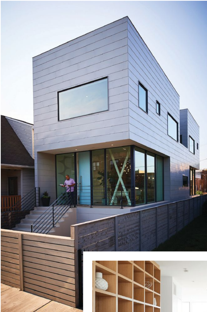
ABOVE: VIEW LOOKING NORTHEAST AT THE FRONT ENTRANCE AND SIDE ELEVATION CLAD WITH FLUSH MOUNTED INTERLOCKING PAINTED METAL PANELS PHOTO BY BOB COSCARELLI
