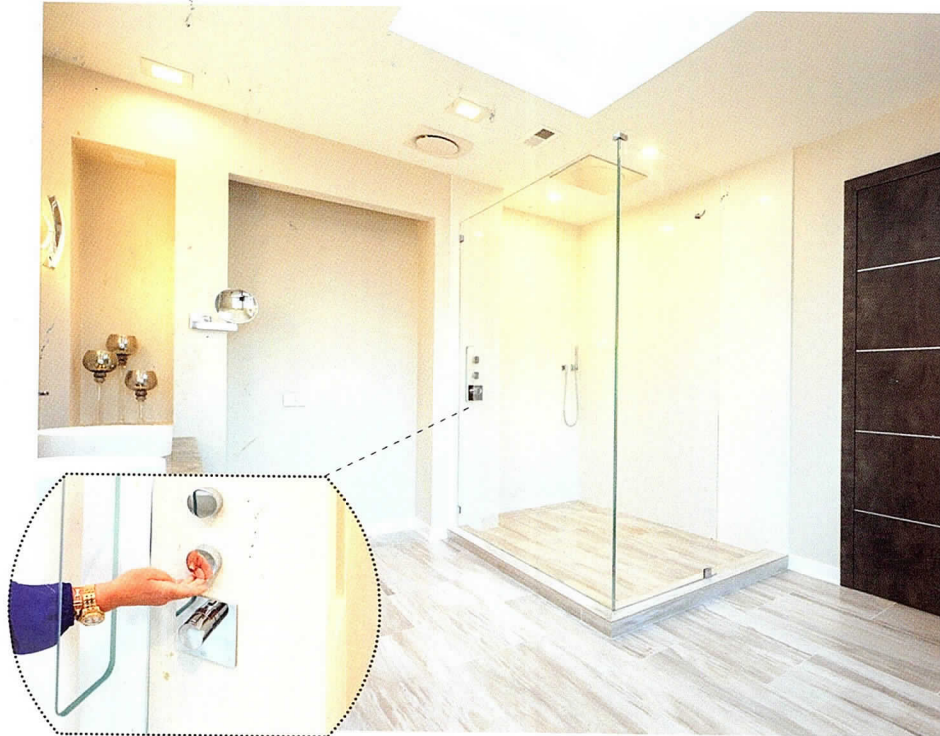
Above: Custom shower. One-half-inch Starphire glass with a custom water jet cutout. Designed by Melissa Garfinkle, InDesign Interiors, Inc.
