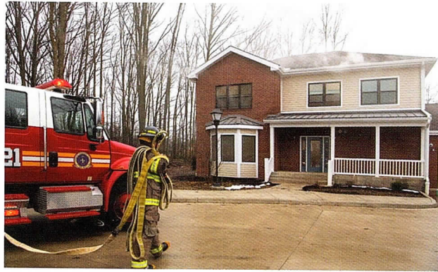
Construction has finished on the Simulated Scenario Village at Cuyahoga Community College's Western Campus (Parma, Ohio). The 40,900-square-foot village, designed by Legat Architects and DS Architecture , offers lifelike first responder training.
