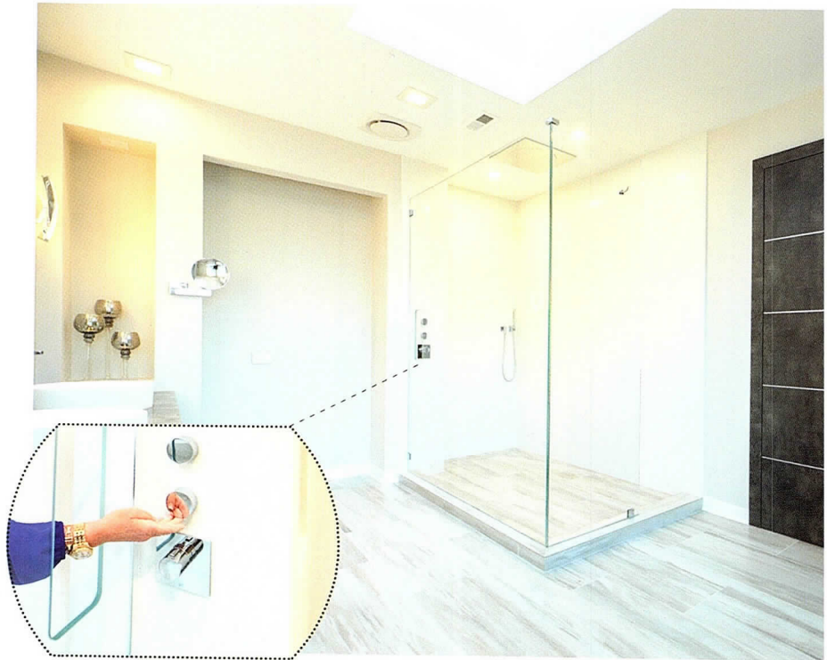
Above: Custom shower. One-half-inch Starphire glass with a custom water jet cutout. Designed by Melissa Garfinkle, InDesign Interiors, Inc.
