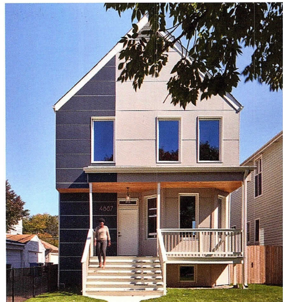
HPZS has designed the first certified single-family Passive House Institute US (PHIUS+) Renovation in Chicago. The objective of this retrofit low-energy project was to bring to market the latest in sustainable homebuilding science in the Midwest in order to transform the speculative renovation market.
