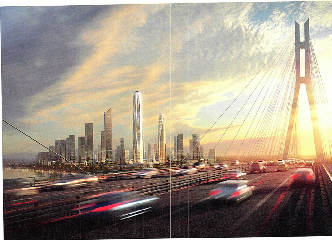
Adrian Smith + Gordon Gill Architecture has released the design of the new South HeXi Yuzui Financial District and Tower. The firm won an international design competition in 2018 to design the new South HeXi Yuzui Financial District and Tower.
