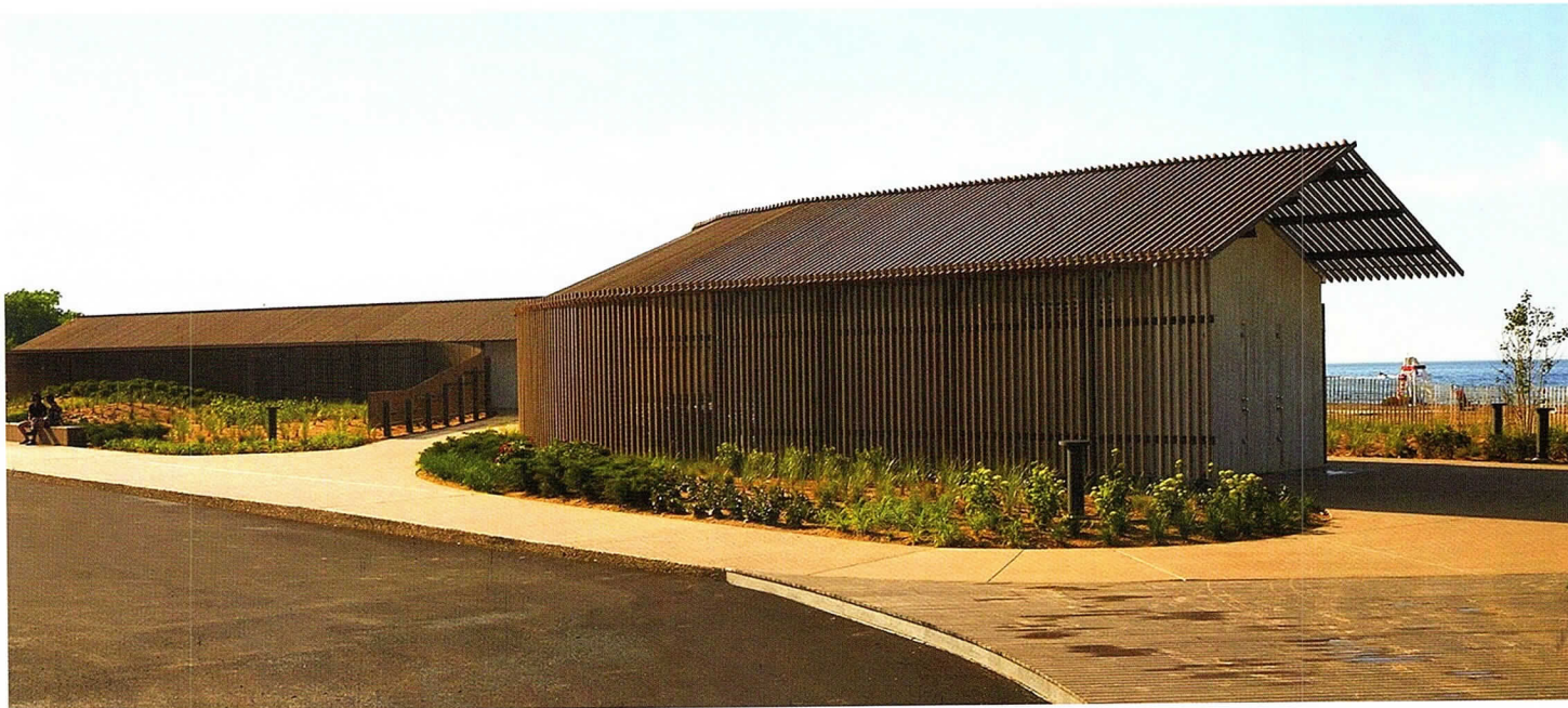
Woodhouse Tinucci Architects received a 2021 AIA national Small Project Award for their Gillson Park Beach House in Wilmette, IL.
