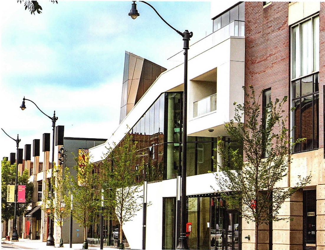
Adrian Smith + Gordon Gill Architecture's new Steppenwolf Theater Art and Education Center will open at the end of the summer. It is the largest permanent cultural asset opening in Chicago this year at 50,000 square feet, including a new 400-seat Round Theater (one of its kind in Chicago), two new bars, and Steppenwolf's first dedicated education center, which will provide programming for teens and the community.
