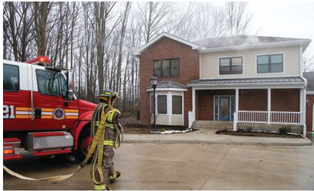
Construction has finished on the Simulated Scenario Village at Cuyahoga Community College's Western Campus (Parma, Ohio). The 40,900-square-foot village, designed by Legat Architects and DS Architecture , offers lifelike first responder training.
