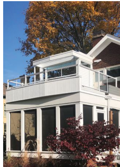
DII Architecture was the architect and builder for a small 1940 home needing a second floor master suite addition, office and green roof deck. The minimalist, sleek addition allows the home's original architectural vernacular to remain intact
