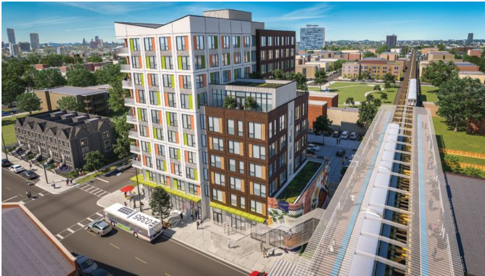
Landon Bone Baker Architects has designed 43 Green, a transit-oriented development comprised of a multiphase, mixed-use, residential and commercial project anchored by the 43rd Street Green Line station at 43rd and Calumet.
