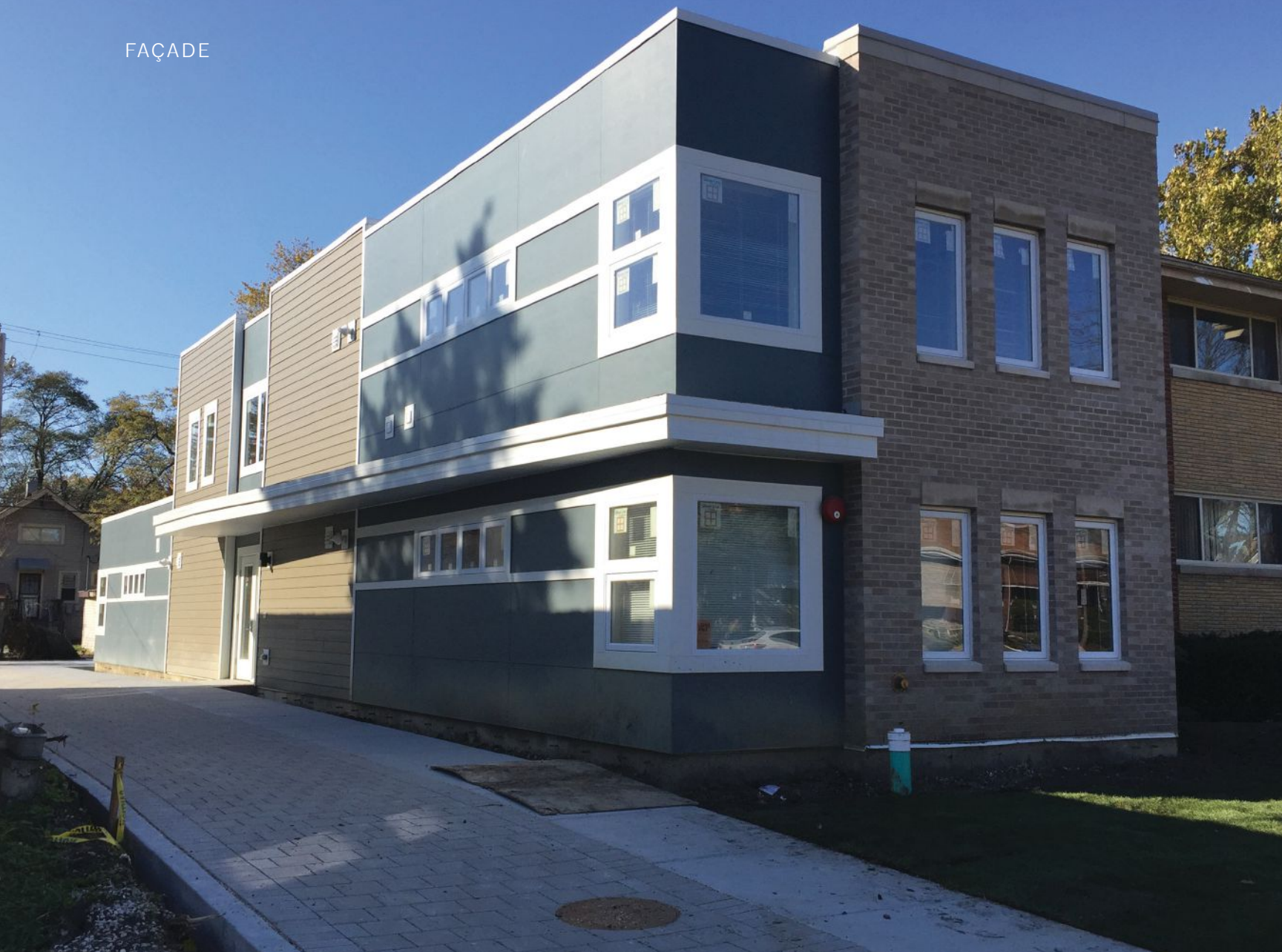
Located in Maywood, this new construction, multifamily home is one of many scattered-site projects called Access West Cook by WJW Architects that integrate highly accessible, transitional housing into residential neighborhoods. ALL PHOTOS BY WJW ARCHITECTS
