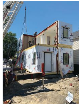
Housing modules are manufactured off-site and are transported and assembled.
