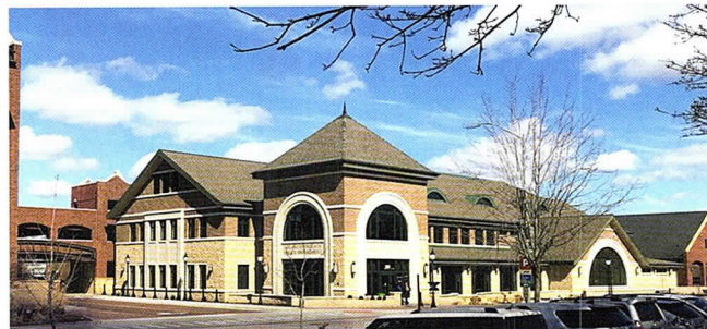
The Village of Arlington Heights Police Station, designed by Legat Architects and built by Riley Construction, has earned a 2020 Project of the Year Award from the American Public Works Association (APWA).
