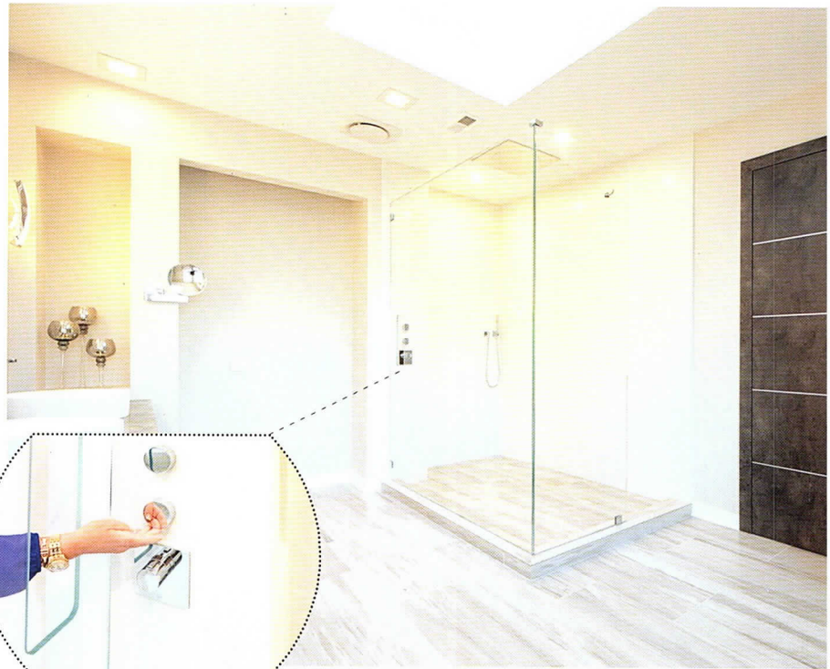
Above: Custom shower. One-half-inch Starphire glass with a custom water jet cutout. Designed by Melissa Garfinkle, InDesign Interiors, Inc.
