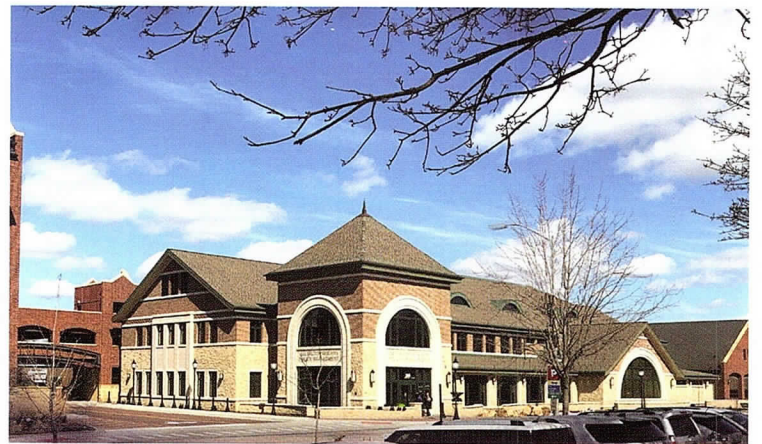
The Village of Arlington Heights Police Station, designed by Legat Architects and built by Riley Construction, has earned a 2020 Project of the Year Award from the American Public Works Association (APWA).
