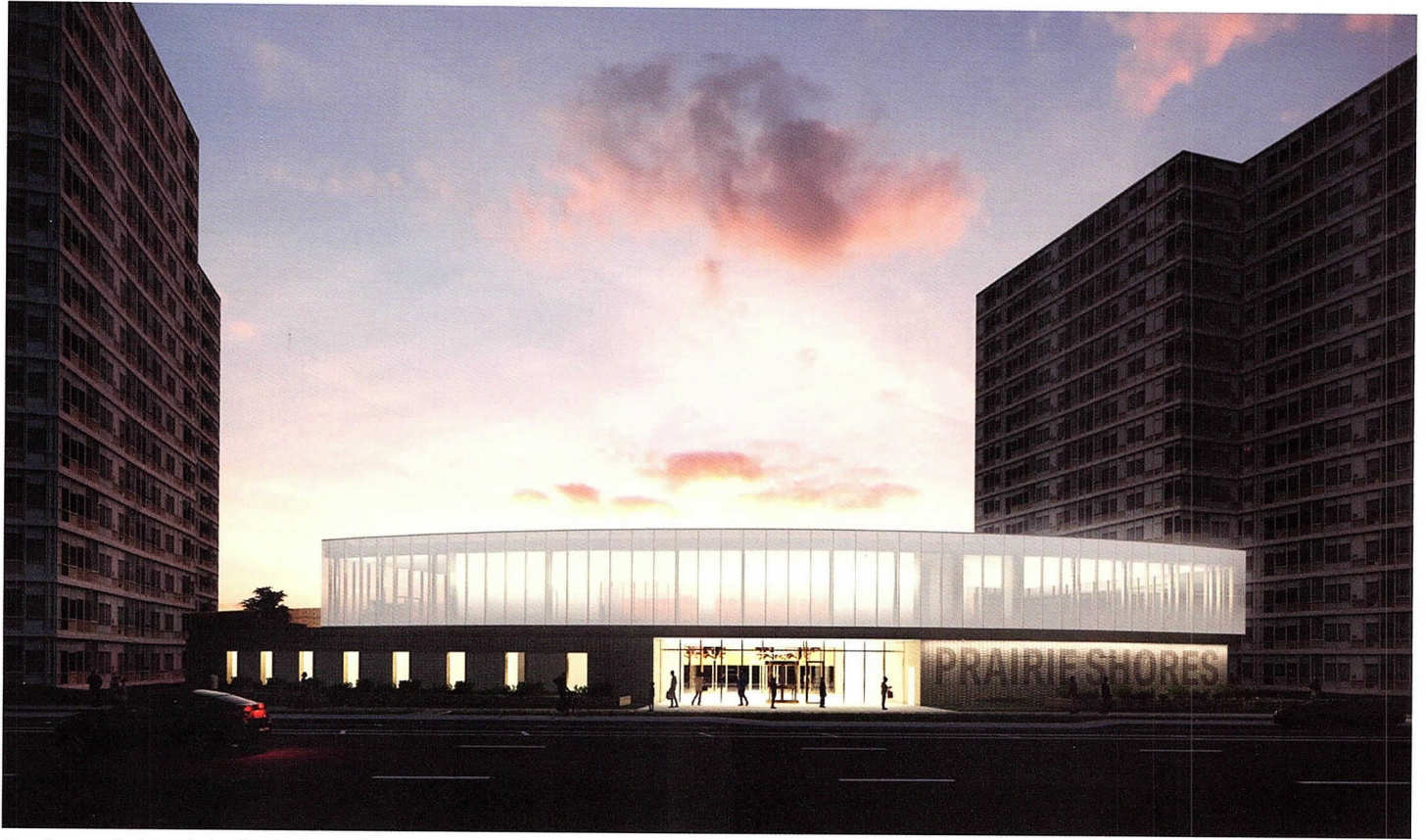
Gensler unveiled the design for the Prairie Shores Apartments amenities clubhouse, with interiors by Stanton Interior Concepts.
