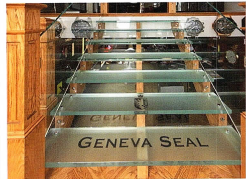
Below: Glass staircase entrance at Geneva Seal Oak Street. 1 1/2-inch tempered, slip-resistant laminated glass with etched, painted lettering.
