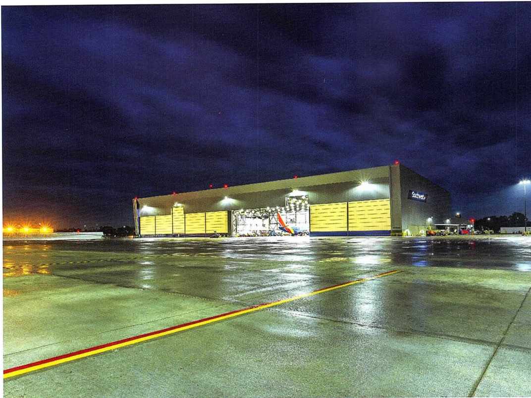
Ghafari Associates recently completed Southwest Airlines' Aircraft Maintenance Center at Houston Hobby Airport — the largest hangar in the airline's network.
