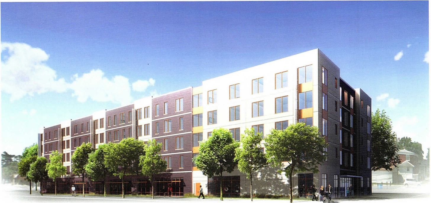
HED recently broke ground on the Fifth Avenue Apartments, a 72-unit affordable housing development on Chicago's West Side.
