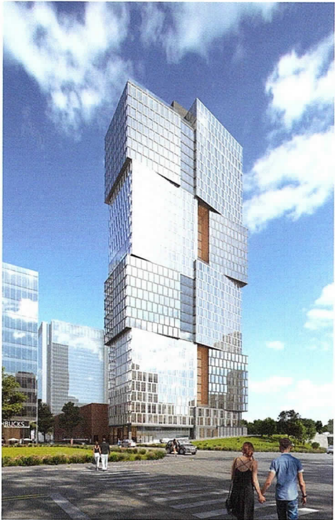
Goettsch Partners has designed Alcove, a new 34-story residential tower in Nashville, Tennessee.
