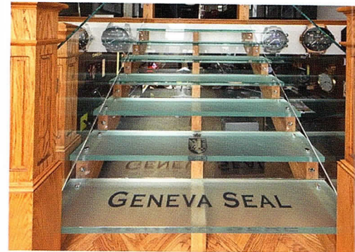
Below: Glass staircase entrance at Geneva Seal Oak Street. 1 1/2-inch tempered, slip-resistant laminated glass with etched, painted lettering
