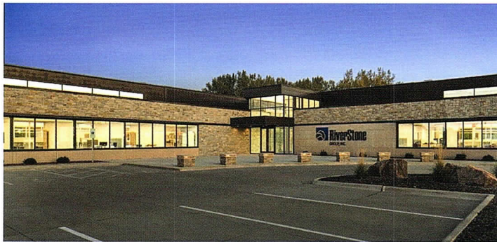
Legat Architects designed RiverStone Group's new 24,000-square-foot headquarters in Davenport, Iowa. The competition-winning design pays tribute to the company's 125-year legacy and to the aggregates that it quarries.
