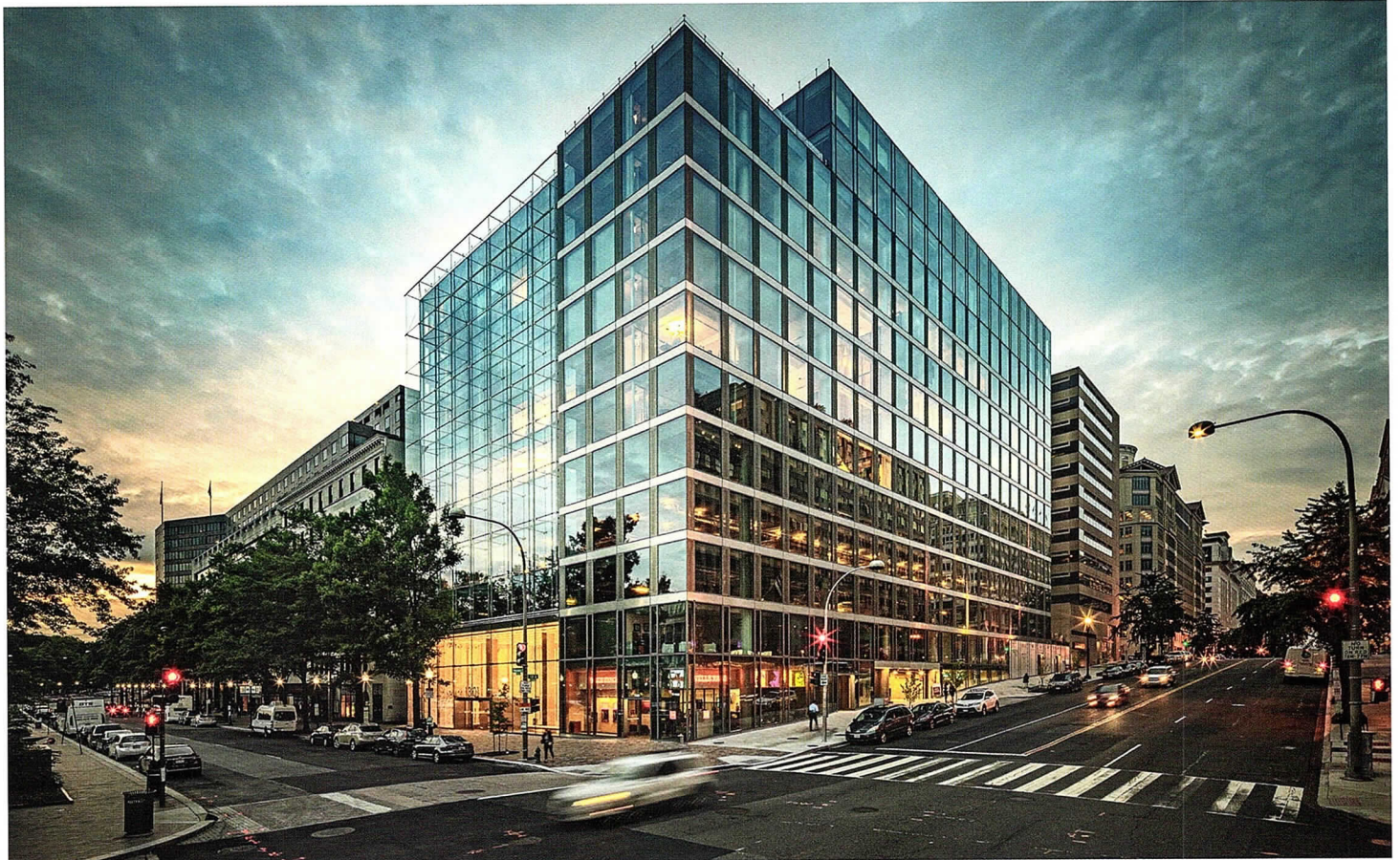
JAHN has completed 1301 Pennsylvania Avenue in Washington, D.C. Of the many sustainable features in this 300,000-square-foot office building, operable windows are provided for all offices within a stainless steel and glass façade. The building is the D.C. headquarters of Kirkland & Ellis.
