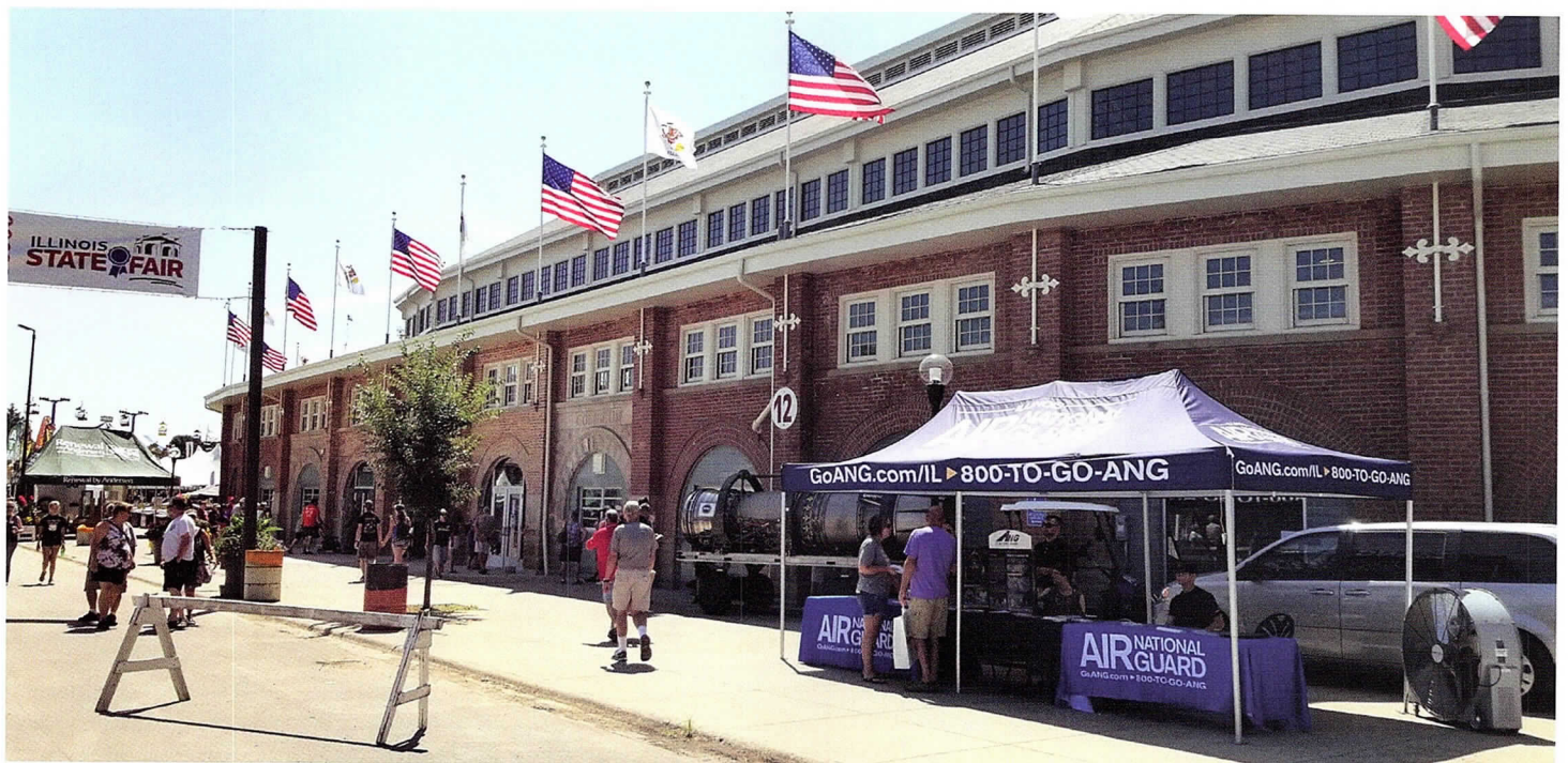
Bailey Edward Design, Inc., has completed Phase I of the renovations of the Illinois State Fair Coliseum.
