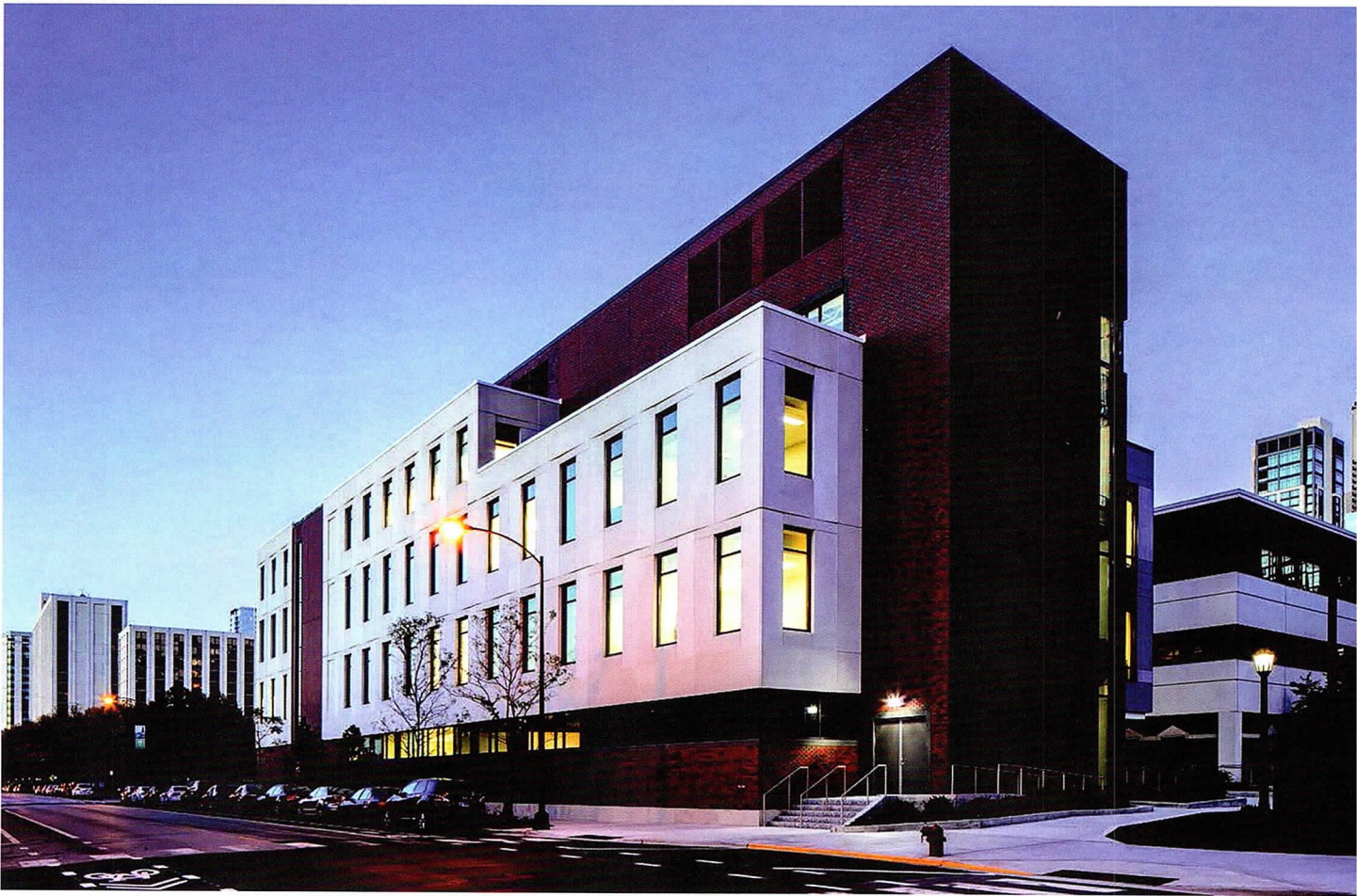
Shive-Hattery has designed the Moody Bible Institute Chapman Center, a new communications center that brings together Moody Radio and Moody Publishers under one roof.
