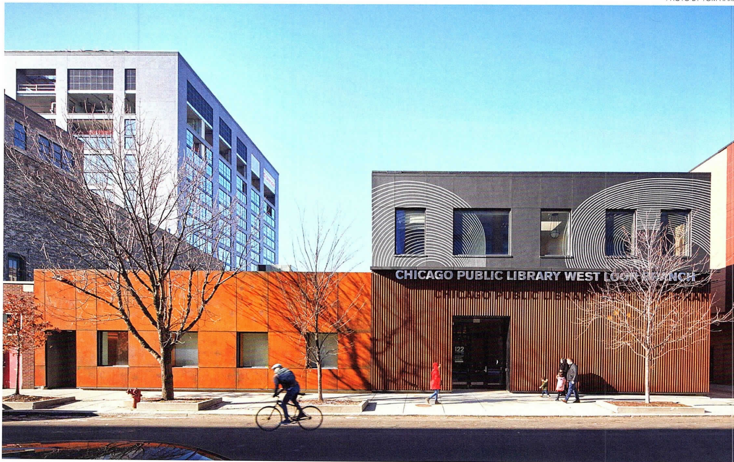
The new West Loop branch of the Chicago Public Library opened in January. Designed by Skidmore, Owings and Merrill LLP , this is the first CPL branch in the neighborhood
