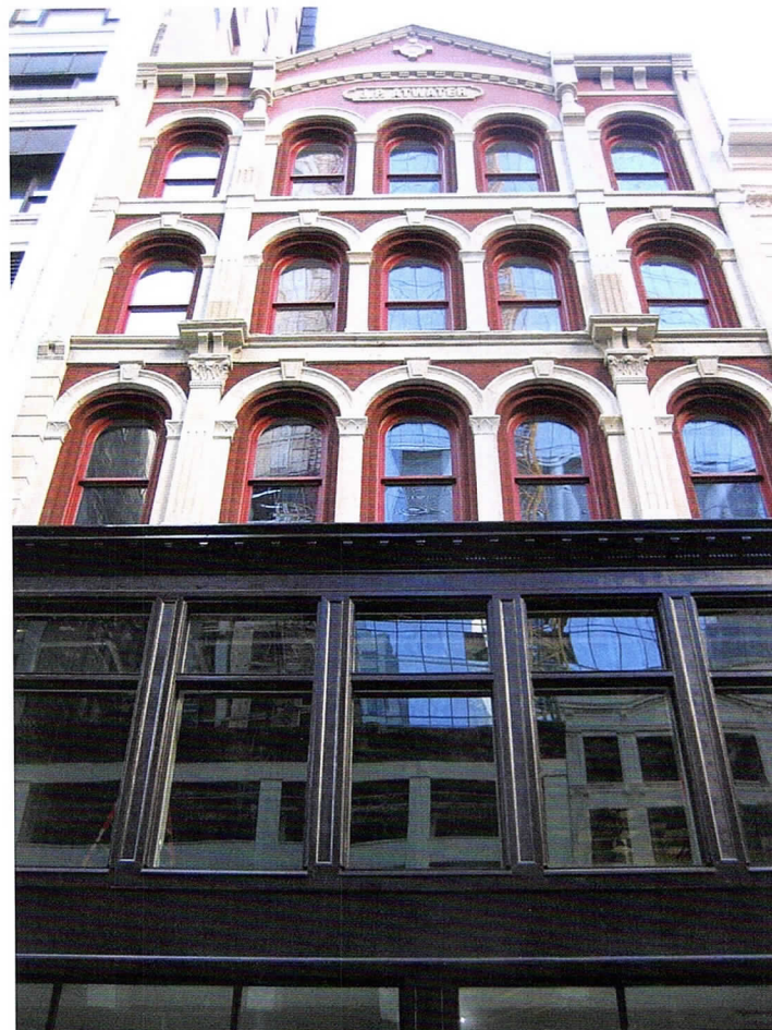
THE ATWATER BUILDING (AFTER RESTORATION) BY HARBOE ARCHITECTS.
