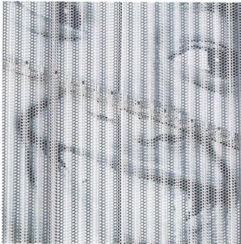
7/8-in. perforated corrugated panels overlay the graphic
