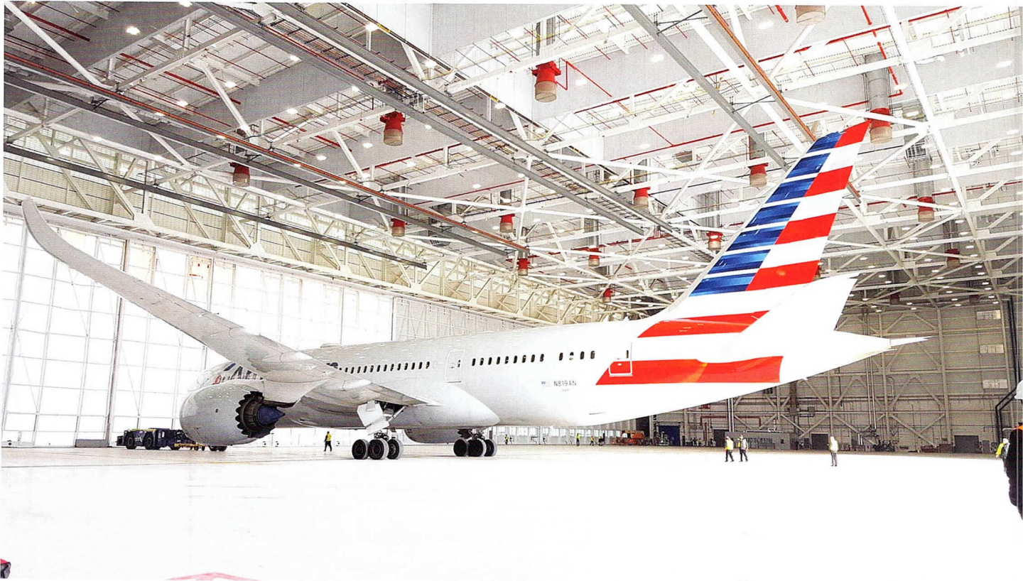
American Airlines will soon unveil its new 194,000-square-foot, double wide-body aircraft maintenance hangar, designed and engineered by Ghafari Associates.
