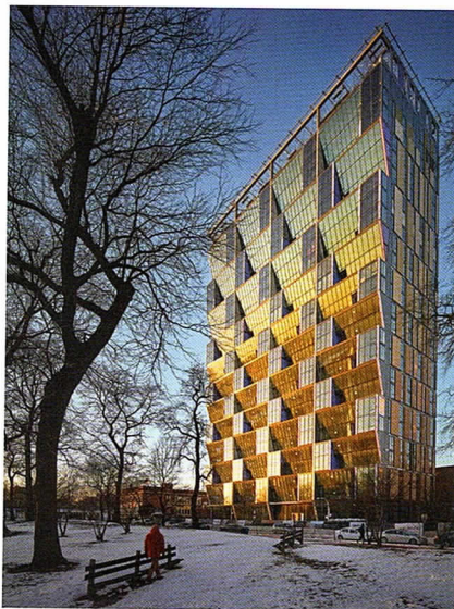
Studio Gang has completed Solstice on the Park, the latest collaboration between MAC Properties and the firm. The residential tower provides self-shading in summer and increased solar exposure in winter months.
