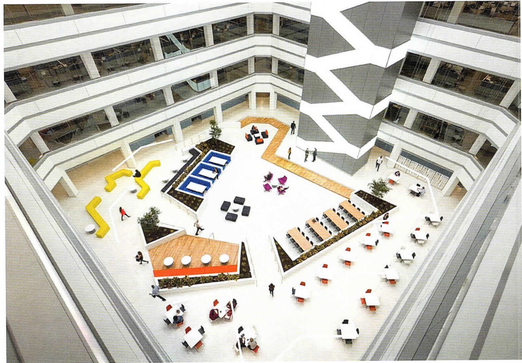
Exp has just completed a major renovation and office realignment at the Charles F. Prevedel Federal Building. Work included site master planning and implementation, renovation of five floors of offices for various federal agencies, and a major redesign of public spaces, including the entry lobby, atrium and café.
