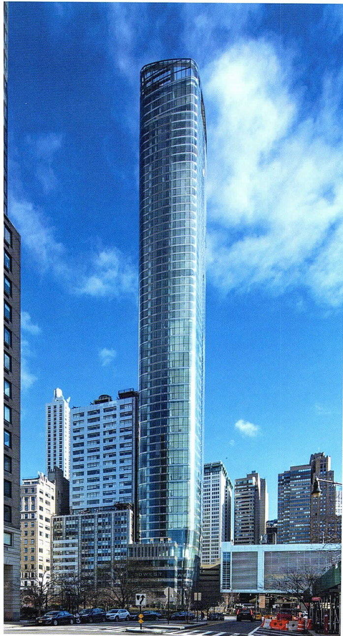
HN's 50 West St. in lower Manhattan was completed in early 2018.
