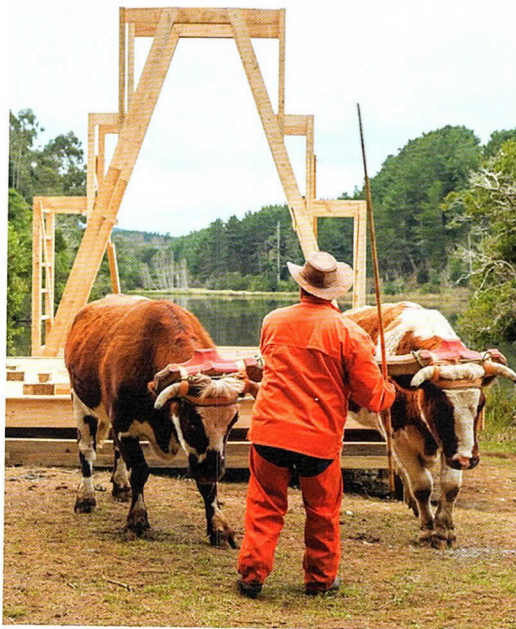
LOCAL OXEN ASSISTED WITH CONSTRUCTION
