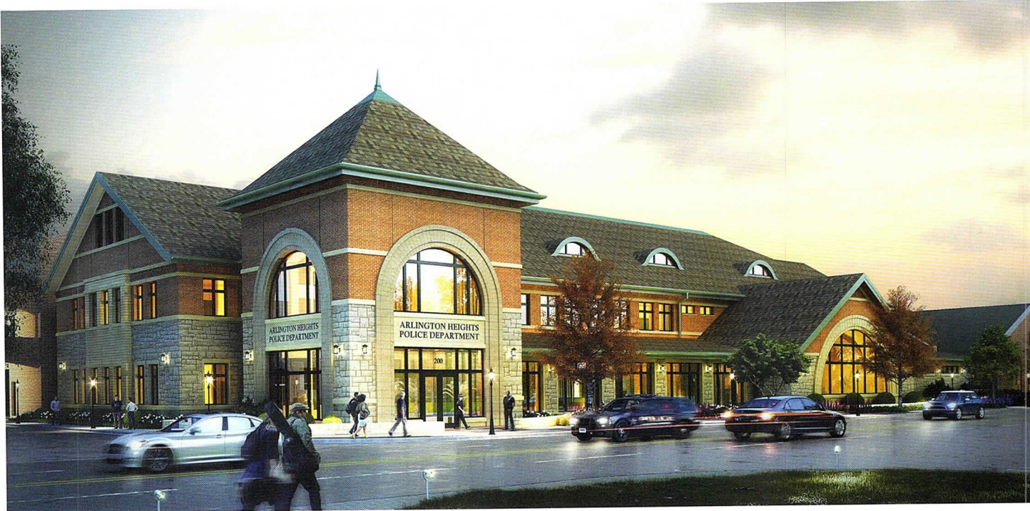
The new Arlington Heights Police Station now under construction was designed by Legat Architects .
