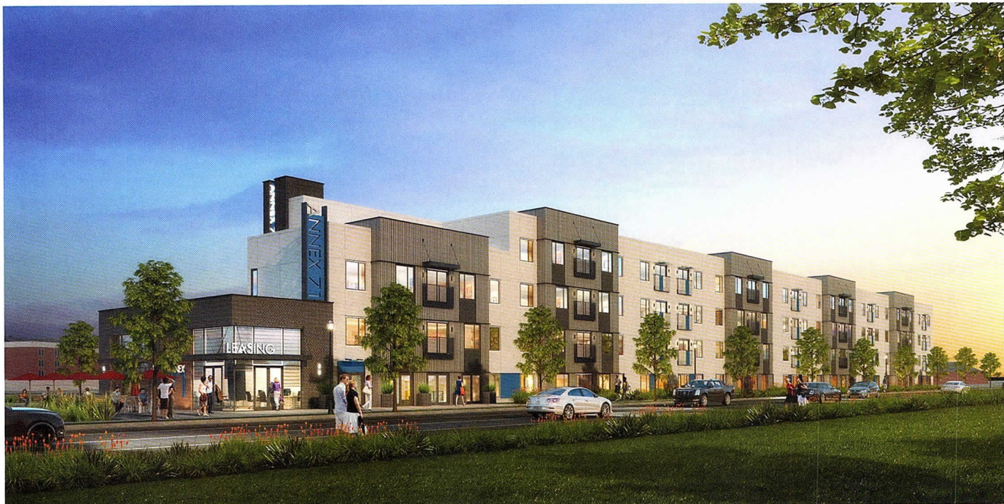
Construction has begun on KTG Architecture + Planning's project, Annex 71. The residential project will create 140 new residences at the University of Wisconsin-Oshkosh.
