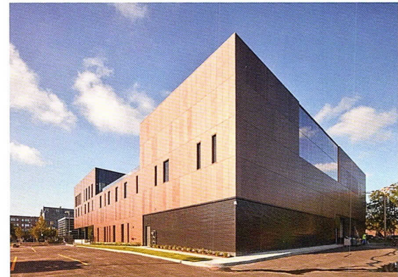
The Gensler-designed, West Loop-located Chicago Plumbers Local 130 Joint Apprenticeship Committee Training Facility showcases advanced water conservation technologies complemented by hands-on labs and classrooms.
