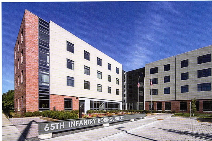
The 65th Infantry Regiment Borinqueneers Veteran's Apartments by Pappageorge Haymes Partners and the Hispanic Housing Development Corporation has been recognized with the Vision Award by the Urban Land Institute Chicago.
