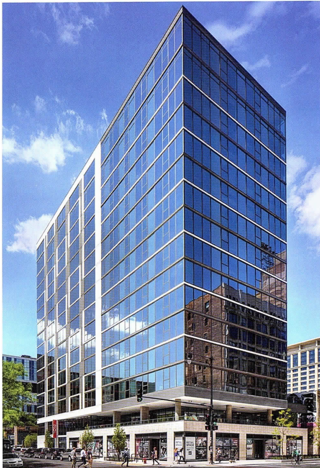
Solomon Cordwell Buenz's "30 East," a brand-new, fully furnished apartment community designed for students and young professionals in Chicago's South Loop, recently opened. The 16-story, 148,000-square-foot building provides 254 beds within 134 apartment units.
