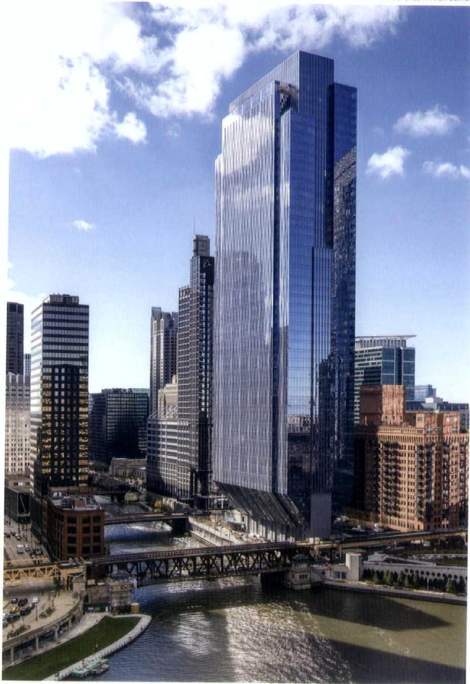
Goettsch Partners -designed 150 North Riverside project opened to the public in April. The 54-story structure features a signature narrow base, which accommodates nearby transit lines and yields column-free floors.
