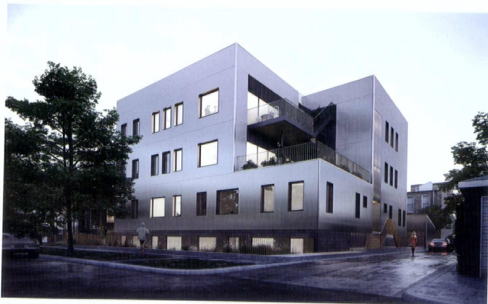
Vladimir Radutny Architects has begun construction on its West Rice Street project. Located in Ukrainian Village, the multi-family unit is distinguished by a corrugated metal skin.
