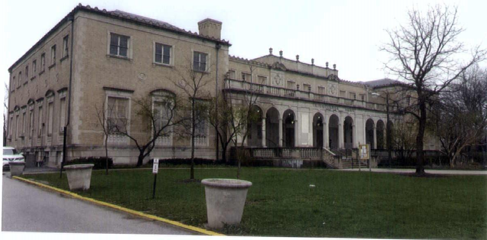
Bailey Edward has been awarded contracts for renovations to six Chicago Park District buildings, four of which are historic. The scope of the projects includes renovations and repairs for water infiltration issues, roofs, repairs to historic landmark buildings, masonry repairs and ADA accessibility. Pictured: LaFollette Park
