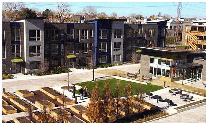
Liberty Gardens Apartments, designed by Landon Bone Baker Architects, opened in Chicago's Near West Side. The new sustainable, mixed-income community offers 76 apartments in seven three-story buildings, and it is organized around a large internal courtyard with green features and amenities, community gardens and gathering spaces.
