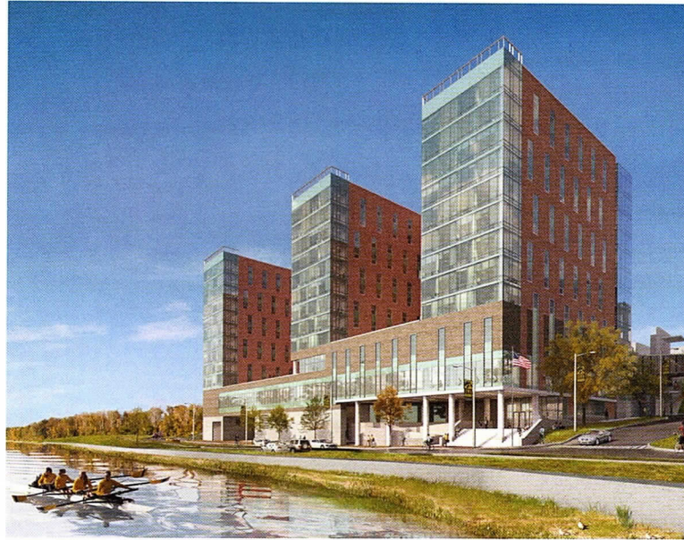
HED recently served as the design architect on the Elizabeth Catlett Residence Hall, a new residence hall at the University of Iowa campus. The hall opens this fall.
