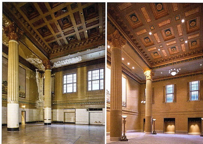
The former Women's Lounge required extensive restoration to nearly every element. The murals had been damaged by both age and humidity. Three of the four murals were restored, while the fourth was recreated by an intricate process of matching digital photograph squares and strips. The alcoves on the far wall formerly served as phone booths.
