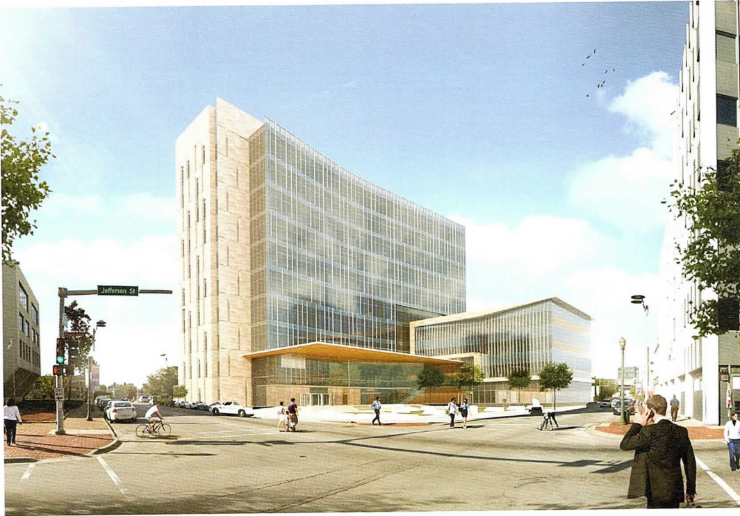
Wight & Company announced its latest project, the Will County Justice Center in Joliet, which will break ground in the spring of 2018. This new center will replace the aging adjacent structure with a modern justice facility featuring modernized security screening, courtroom technologies, energy management and sustainable design strategies.
