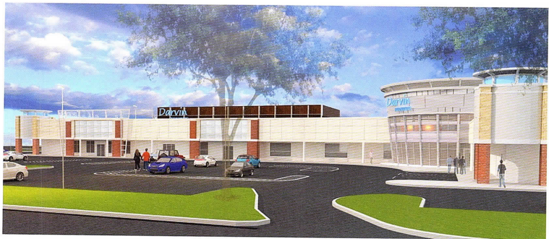
Architectural Resource Corporation (ARC) has designed façade renovations for Darwin Furniture in Orland Park, Illinois. The project includes a new entry node to improve visibility from LaGrange Road and daylight and define the entry; and stainless-steel metal-mesh screens, new signage, lighting and site improvements.
